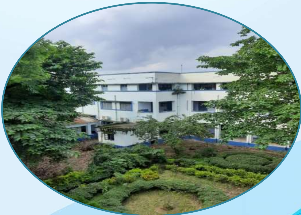
Panoramic view of College building
